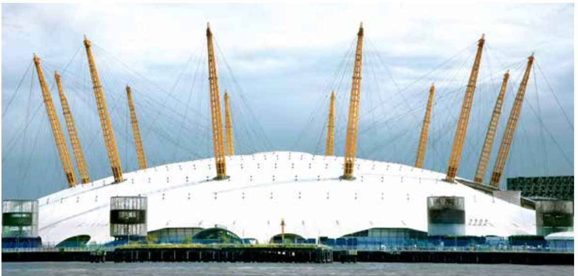
O2 Arena London (UK) – Arch. Richard Rogers
